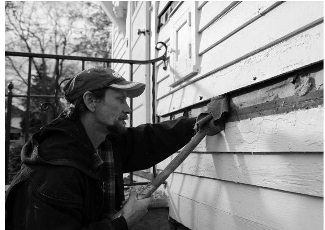
Installing sidewall blow-in insulation.
